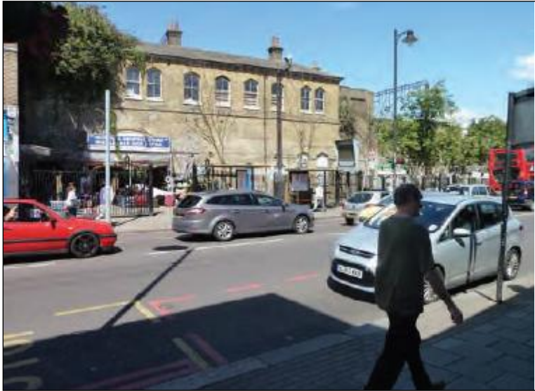
Existing site looking north
